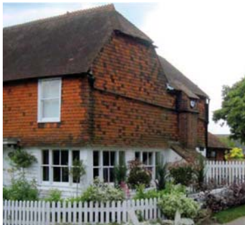
Hipped roof ends
